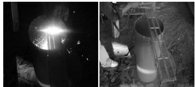
Fig.3. Openings cut by Plasma cutting machine
